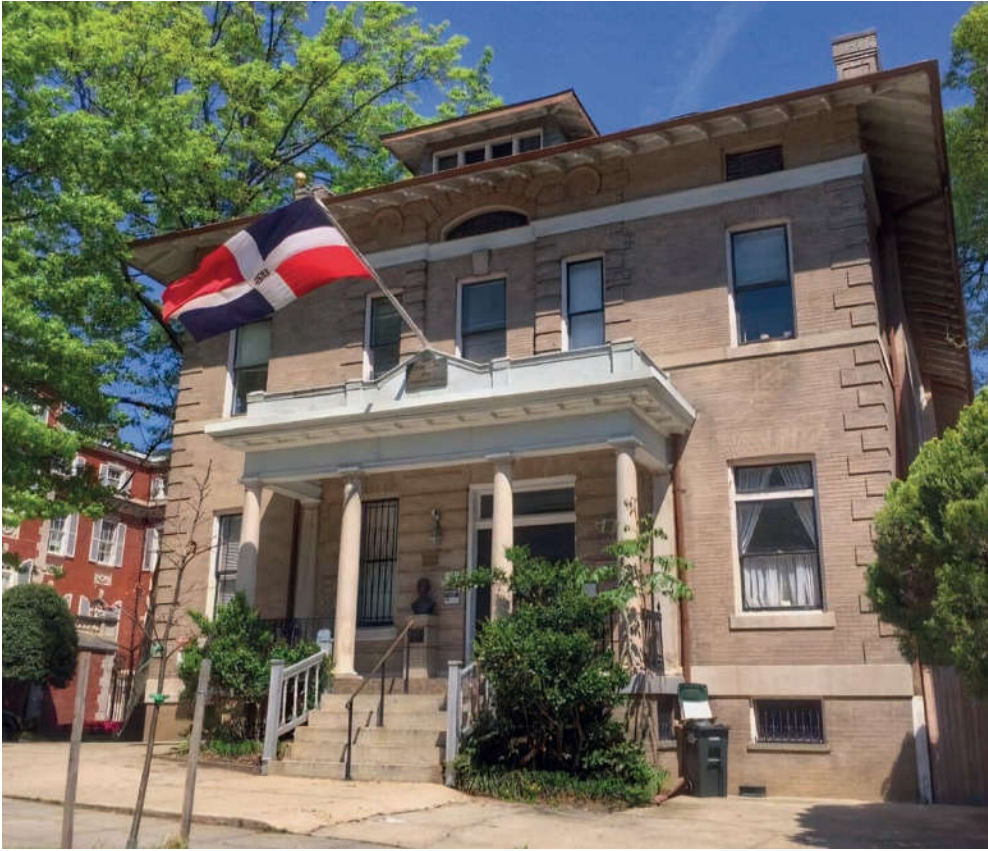
Façade of the former Belgian chancery at 1715 22 nd Street, 2020 (Image provided by the Embassy of the Dominican Republic in Washington, D.C.).
